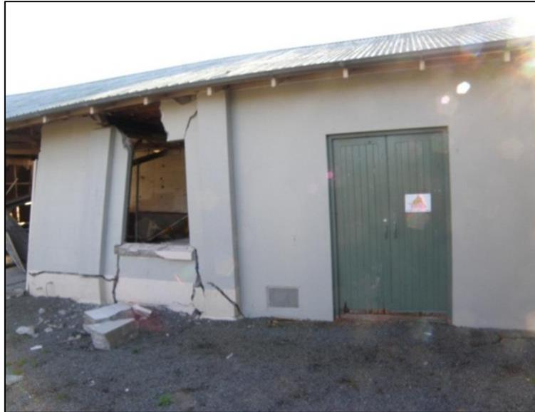
Figure 5 - Redcliffs waterworks substation in Christchurch - Orion had strengthened the right-hand side of the Building<sup>15</sup>
