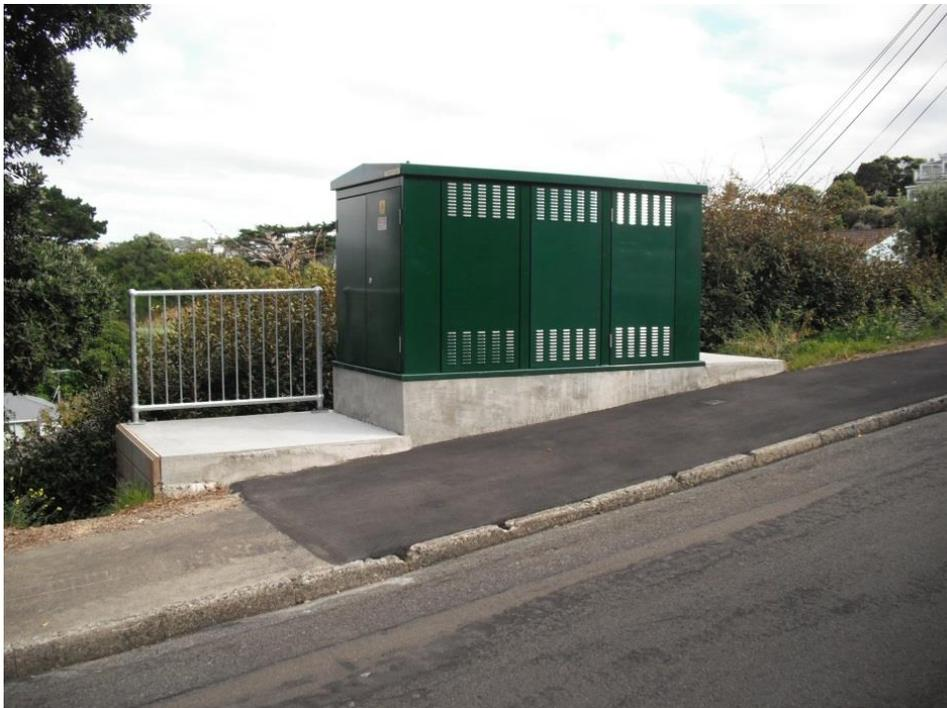
**Photo of a Berm Distribution Substation**
