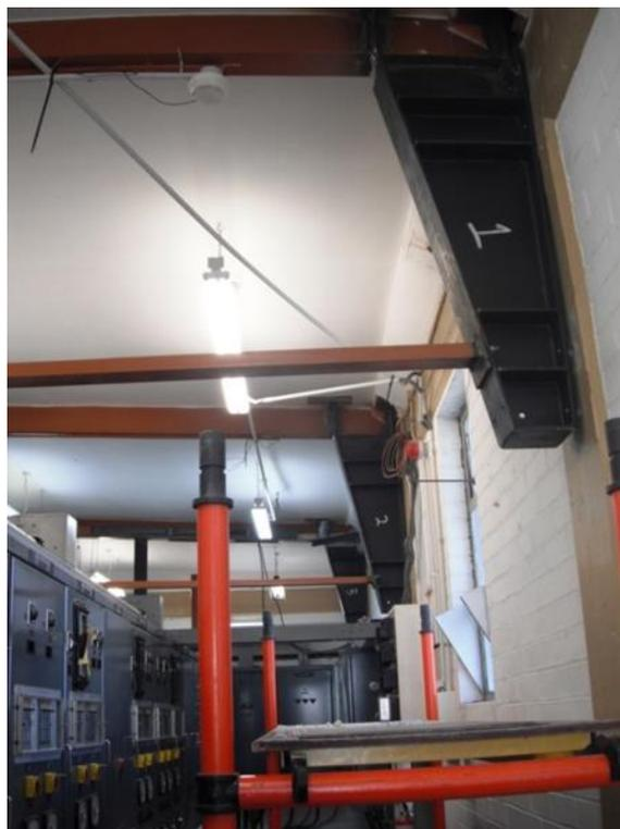
Figure 5-14 Seismic Strengthening at Gracefield zone substation
