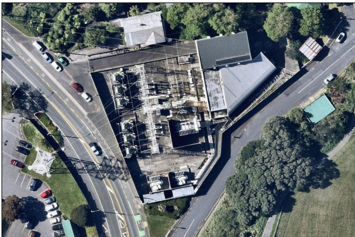
Figure 12-3 Central Park Substation
