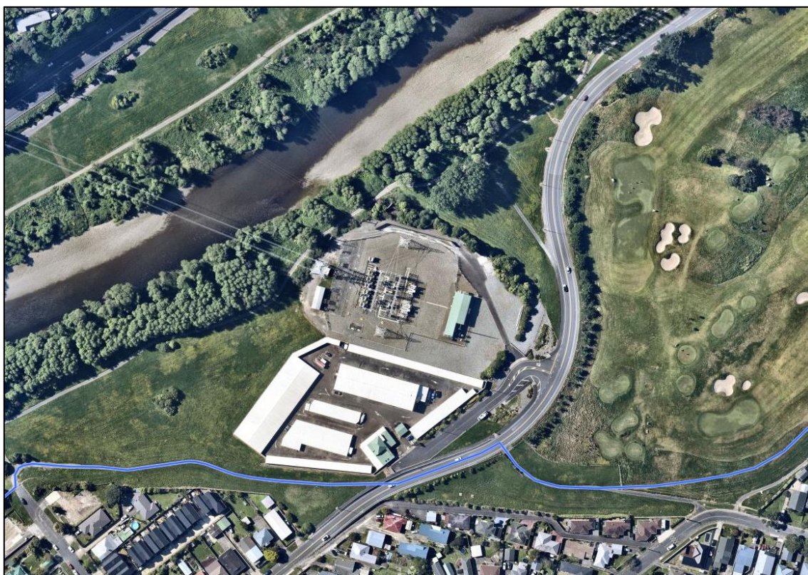
Figure 12-4 Melling Substation (Hutt River stop bank location shown in blue)
