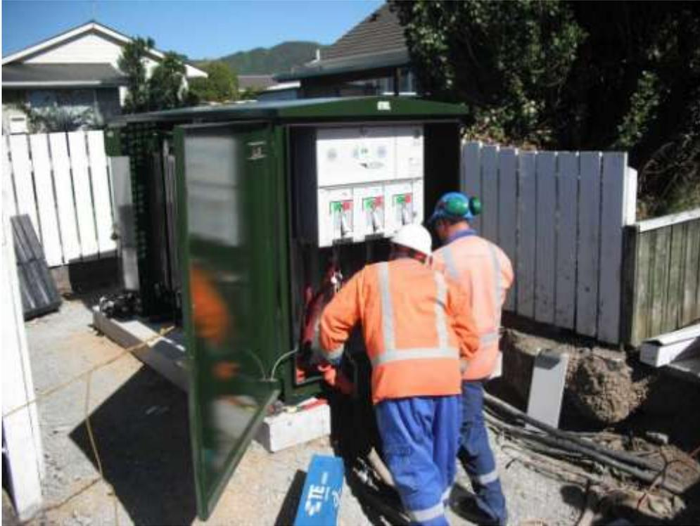
**Installation of a replacement distribution substation**
