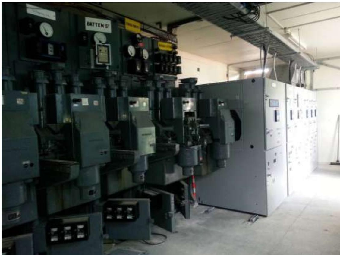
Replacement in progress of Reyrolle Type C with RPS LMVP switchgear at a zone substation
