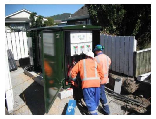
Installation of a replacement distribution substation
