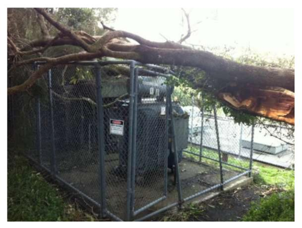
A distribution substation damaged by a fallen tree following a storm
