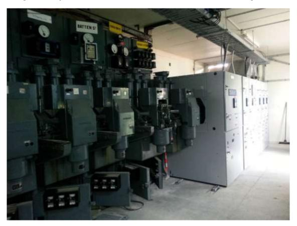
Replacement in progress of Reyrolle Type C with RPS LMVP switchgear at a zone substation
