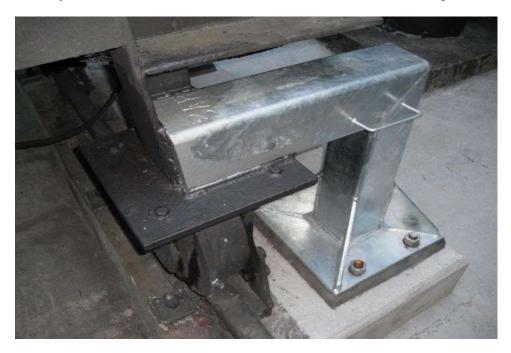
Figure 8-17 Zone Substation Power Transformer Seismic Restraint Footing
