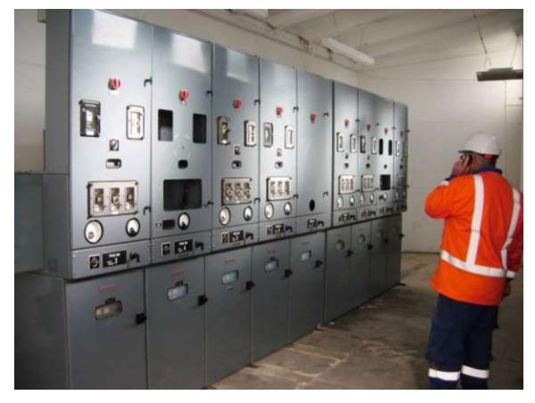
Typical installation of Reyrolle LMT switchgear at a zone substation
