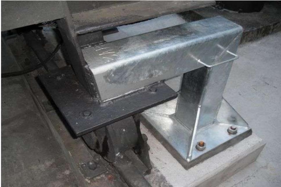
**Figure 8-17 Zone Substation Power Transformer Seismic Restraint Footing**
